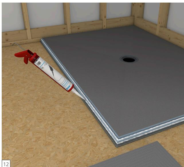
**EN** A  $\frac{1}{2}$ " bead of wedi joint sealant is continuously applied on the horizontal and vertical surface area of the Fundo base channel.
