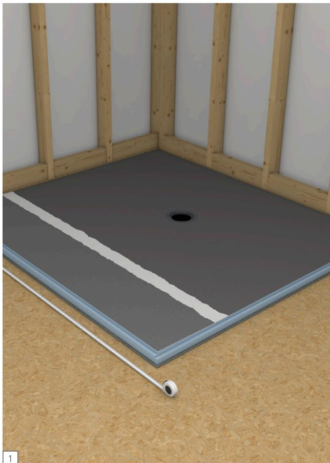
**EN** Determine measurements for the next extended shower area. In this example, we are extending the shower area in one direction only using our extension panels to connect to a previously installed extension panel. In this way, wedi Fundo shower bases can be extended indefinitely. Please note that all added extensions will increase the height of the construction from the floor through the slope built into the extensions.
