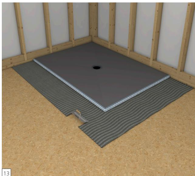
**EN** Apply a modified thinset bed on the subfloor as well as on the underside of the extension using a  $\frac{1}{4}$  in. x  $\frac{1}{4}$  in. square notch trowel on each surface. Make sure the mortar does not contaminate the joint sealant.
