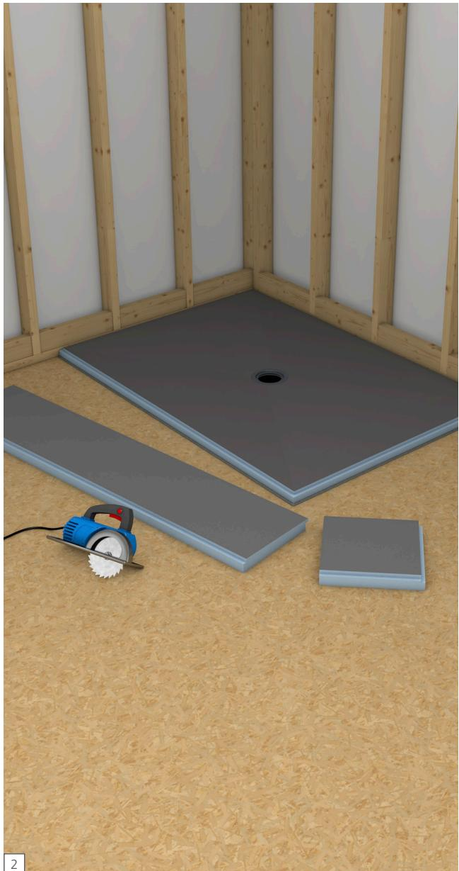
**EN** Cut the extension panel to size using a circular saw or handsaw and dry-fit the extension panel to the shower base's perimeter channel. wedi Extensions should never be cut to a size smaller than 3 inches in length in direction of slope in surface. The extension panel features pre-made channels 1/2 in. deep and 1/2 in. wide, to connect to the shower base, as well as channels on its top surface perimeter where wedi Building Panels (at a wall transition), or a curb can be connected safely.
