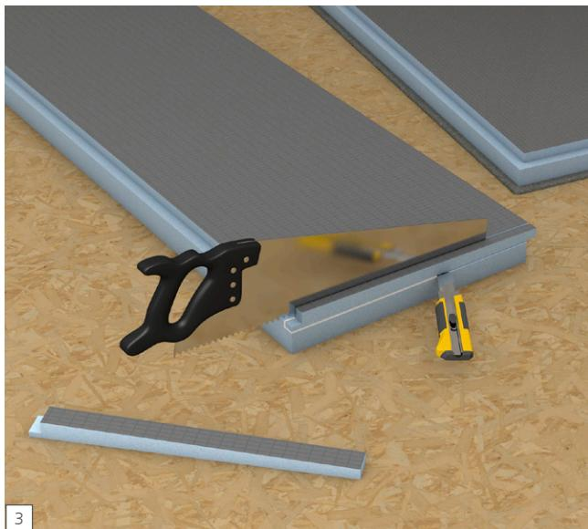
**EN** If additional channels are needed after cutting to size, these can be re-made and cut out using a circular saw and/or a utility knife.
