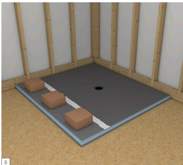
**EN** Weights are applied equally over the shower floor to promote a firmer bond with the thinset mortar allowing you to continue working on the shower walls immediately.
