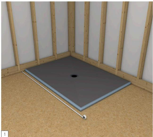
**EN** wedi Fundo shower base is installed first. Determine measurements for the extended shower area. In this example, we are extending the shower area in one direction only using our extension panel.
