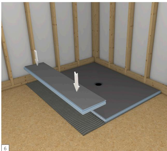
**EN** Install and press the extension panel into the thinset bed and let it connect tightly into the channel connection of the Fundo shower base. Use a flat putty knife to spread all excess joint sealant flat over the connection seam.
