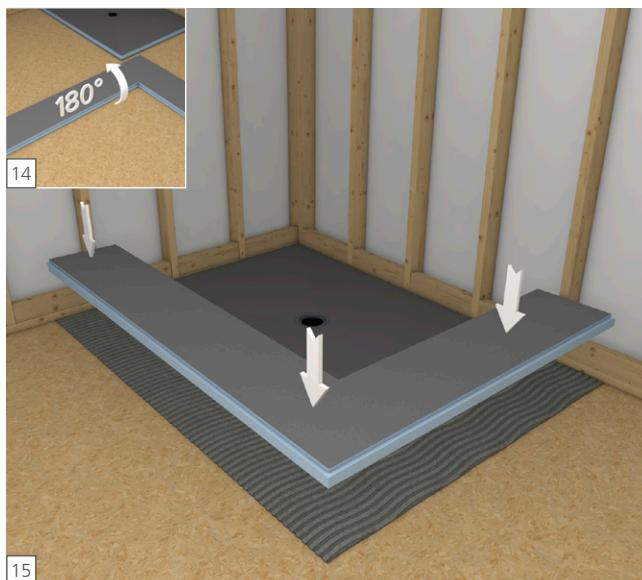
**EN** Carefully turn the extension panel corner so its sloped side is up. Press the panel firmly into the thinset bed.
