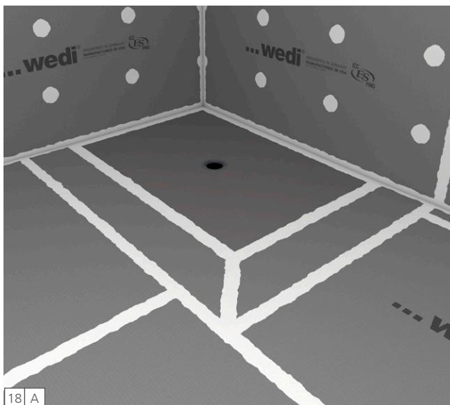
[EN] The installation can now be completed using wedi Building Panel for walls and bathroom floor.
