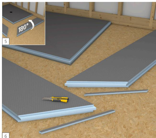
**EN** Turn both extensions on their back and cut a 1/2 in. x 1/2 in. notch channel into each extensions edge where both extensions connect. Make and dry-fit a strip of 1/2 in. Building Panel into the 1 in. x 1/2 inch channel formed by the two extensions where these join.
