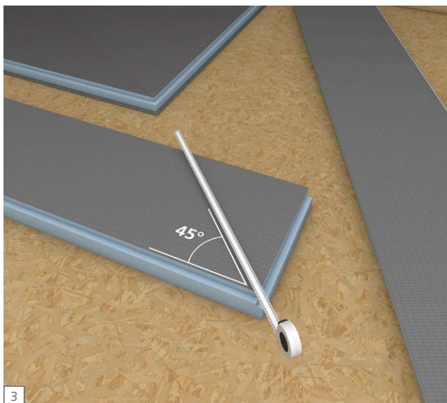
**[EN]** Measure, cut and dry-fit two extensions so they can be abutted along a 45 Degree corner seam.
