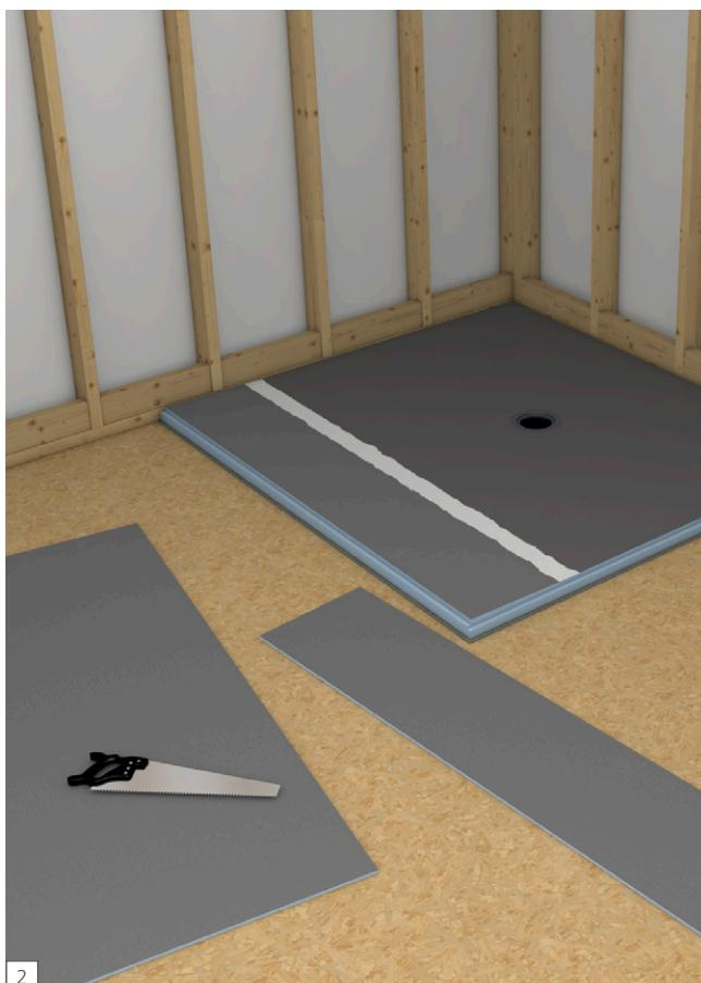
**EN** Usually, this requires adding additional wedi Building panels of the thickness types 1/8 in., 1/4 in. or 1/2 in. to build up the added extension for a tight fit. Panels may need to be combined and multiple panels are adhered using a full surface contact bed of thinset mortar applied using a notch trowel between 1/8 in. square to 1/4 in. square. Please dry-fit this build up and consider the thickness of mortar to be added.
