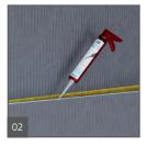
A continuous 1/2" (12.7 mm) bead of wedi Joint Sealant is applied on the foam edges of a wedi Building Panel before another panel is joined by butting tightly.
