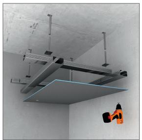
Install the ceiling suspension systems to the existing ceiling by using dowels and set the desired suspension height.
