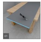
Using only a utility knife, wedi Building Panels are effortlessly cut and shaped.
