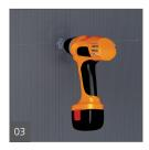
Apply 1 wedi fastener per every 12" (304.8 mm), with an extra fastener applied directly in the seam to provide a flush transition between panels. On a ceiling, apply 1 wedi fastener per every 6" (152.4 mm). The washer heads are dimpled below the surface of the wedi Building Panel so a flat surface is maintained.
