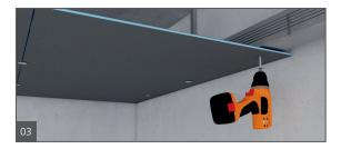
Screw wedi Building Panels to framework using wedi's ceramic coated coarse thread screws and galvanized tab washers. Self tapping screws will be need when installing to metal framing 18 ga. or heavier. The fastener pattern is 1 fastener per every 6" (152.4 mm). Make sure to always use washers/fasteners in panel seams to ensure smooth transitions.
