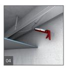
When installing wedi Building Panels to metal stud ceiling framework, use wedi Joint Sealant in addition to wedi screws and Washers.
