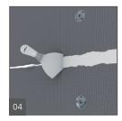
All excess wedi sealant is spread flat over all joints using a putty knife. Where needed, an extra bead of sealant is applied on top of the joints and spread flat. The joints should be covered a full 1" (25.4 mm) on both sides of the seam. Especially wedi Joint Sealant provides little build-up making for square and tight corner areas perfect for tiling. All fastener locations are waterproofed using wedi Joint Sealant spread flat and widely over each washer.
