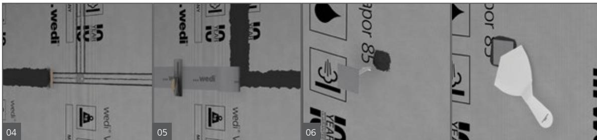
4. Apply several beads of wedi Sealant 620 as a setting and sealing bed for wedi sealing tape. Spread the sealant with a fine tooth adhesive trowel or flat putty knife to achieve a full coverage sealant bed for the sealing tape. The minimum thickness of the sealant bed should be 1/16 in. (1.5 mm).
