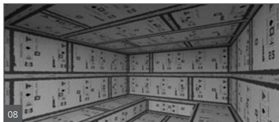
8. Allow the wedi Sealant 620 to cure for at least 24 hours prior to setting tile and 96 hours after its application before exposing the tiled installation to water and water vapor. On floor areas, consider wedi Fundo Shower Systems or Subliner Dry sheet waterproofing membrane when working over mortar or screed surfaces (install in accordance to Subliner Dry installation manual using wedi Sealant 620 in overlapping sheet – or Subliner Dry tape covered seam connections).
