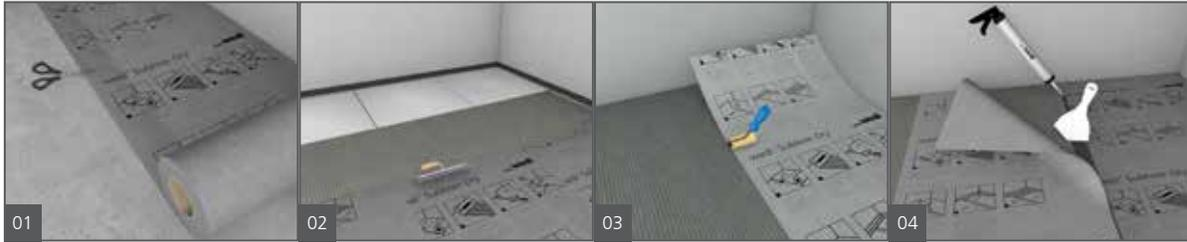
1. Lay out wedi Subliner Dry and cut to size using a knife or scissors.
