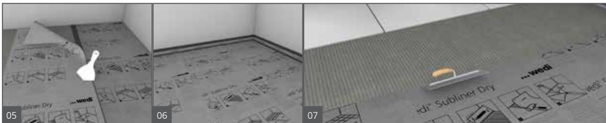
5. Spread the wedi Sealant 620 flat using a putty knife. Cross joints should be avoided.
