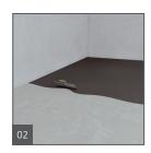
The panels are installed in a full coverage setting bed using modified thinset mortar allowing best connection between subfloor and wedi Building Panel.
