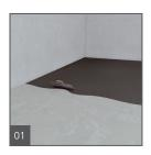
Make sure the concrete floor is even, fully cured and free of debris, oil or waxes. The wedi Building Panels are installed using modified thinset mortar using a 1/4"  $\times$  1/4" (6.4  $\times$  6.4 mm) notch trowel.
