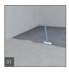
Make sure the concrete floor is fully cured and free of debris, oil or waxes. Some concrete floors might require priming or vapor retarders prior to thinset mortar installation.
