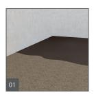
Simply spread modified thinset mortar over a clean wood subfloor using a  $1/4" \times 1/4"$  (6.4  $\times$  6.4 mm) notch trowel provided the subfloor is even and load-bearing.
