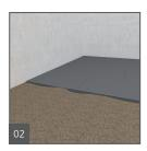
Apply the wedi Building Panel by laying the panels into the mortar. Stagger all panel joints. Apply weights, such as tile boxes, equally across the wedi Building Panel surface and especially over transitions.
