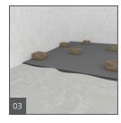
Stagger all joints when laying wedi Building Panels on the floor. Apply some weights such as tile boxes equally distributed over the wedi Building Panel surface and especially over transitions.
