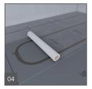
Apply wedi's wide self adhesive reinforcement tape over the installed ducts. You can then start tilling. Tiles smaller than 4  $\times$  4" (101.6  $\times$  101.6 mm) should not be used over hydronic system installation surfaces.
