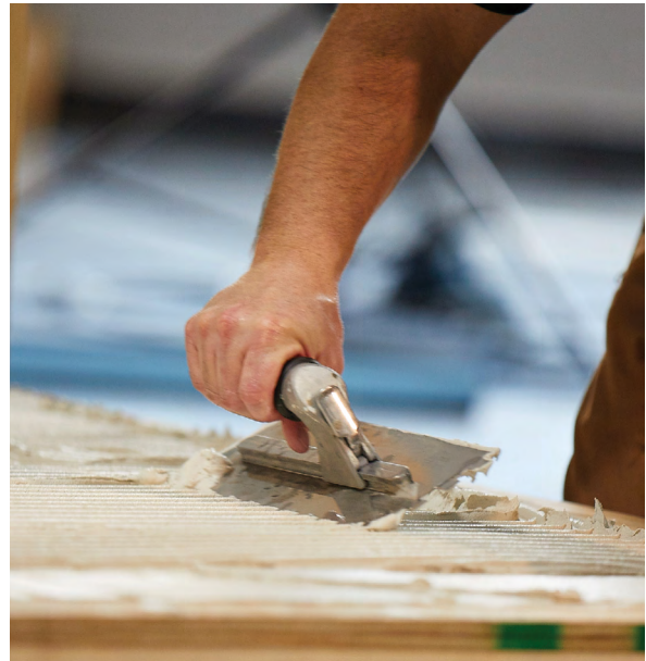
Glass and Stone Tile Installation (see Details for "Cementitious Coated Extruded Foam Backer Board").
