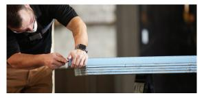
A wedi shower base can be cut to size using a circular saw with standard carbide blade. You can remake the 1/2 inch x 1/2 inch perimeter channel by cutting through the cement surface using the circular saw set to cut 1/2 inch deep. You can use a circular saw or a sharp utility knife to cut the new channel 1/2 inch wide through the blue exposed foam side. Clean the new channel and the base and remove all saw dust and loose particles.
