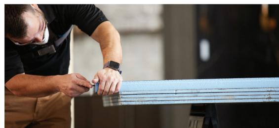
A wedi shower base can be cut to size using a circular saw with standard carbide blade. You can remake the 1/2 inch x 1/2 inch perimeter channel by cutting through the cement surface using the circular saw set to cut 1/2 inch deep. You can use a circular saw or a sharp utility knife to cut the new channel 1/2 inch wide through the blue exposed foam side. Clean the new channel and the base and remove all saw dust and loose particles.
