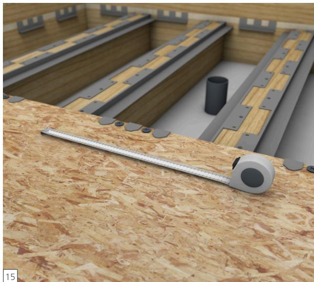
**EN** Measure and mark to cut wood strips tightly fitting into the recess bracket support system between joists, wall framing and regular subfloor. Leave a 1/8" (3.2 mm) gap between wood strips and brackets so the wood may move without creating too much tension.
