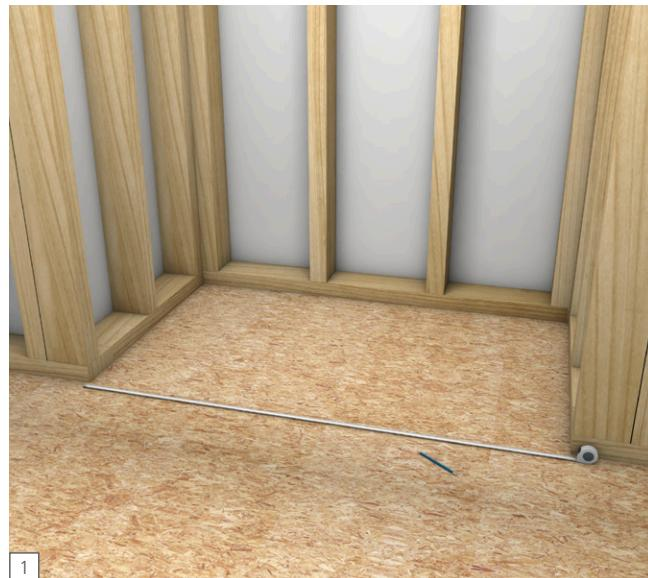
**EN** Measure and mark subfloor to be removed. Use a safe saw to cut close to the framing but also in a safe and clean way. wedi recommends a combination of saws including a sawzall and a saw like Dremel (r) US40 01 120 V where a standard circular saw might not reach.
