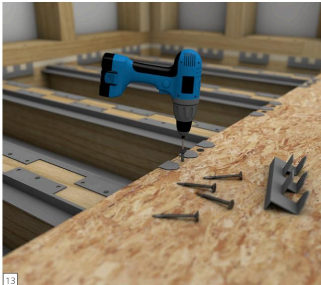
**EN** Use flat head Phillips self-drilling screws with wings provided by wedi to fasten C brackets to the edge of the wood floor plate at the open side of the future shower area. Fit brackets between flanges of joist/wall brackets. Use two (screws) to fasten this bracket through the wood floor and into the lower claws.
