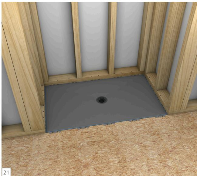
**EN** Your Ligno shower is now flush with the surrounding subfloor and is supported by a subfloor with absolute structural integrity, so important for safe tile installation and without the risk of cracks in tile or grout so typical to tile substrate installations or shower systems installed with insufficient support.
