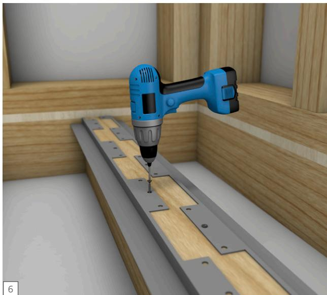
[EN] Repeat process shown under 4. and install joist brackets to all exposed joists.
