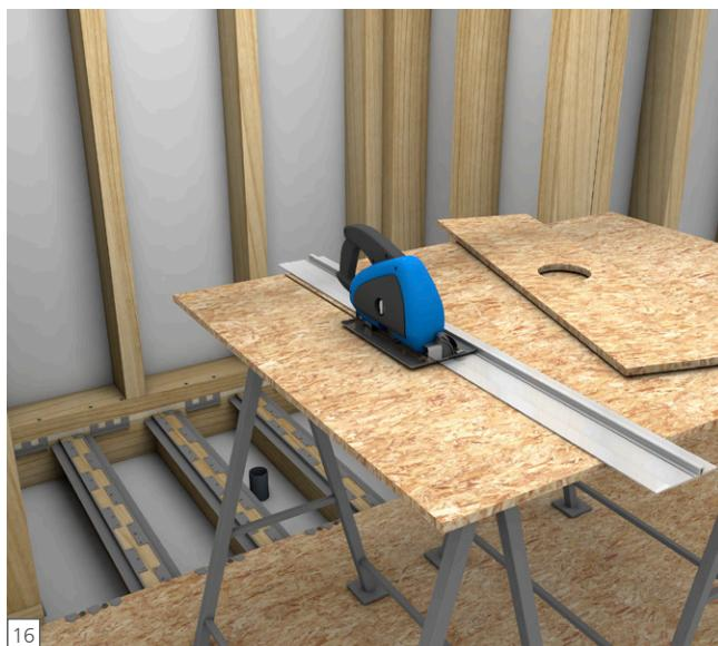
**EN** Cut the wood floor strips incl. the strip for the drain area featuring a 6 1/2" (165.1 mm) diameter hole to be seated over the center of the floor waste pipe.
