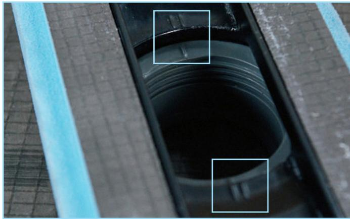
In case it is difficult to hear the click mechanism, on the top side of the base you can also verify the drain unit has successfully connected when the single hash marks are centered between the double hash marks as shown here. Should you want to remove the drain body at any time, this can be done by pushing the snap mechanism's plastic flap inwards using a flat headed screwdriver and unscrewing the Drain Body to the left at the same time.
