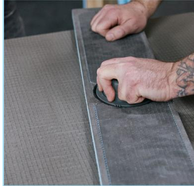
Once inserted, turn the Drain Body clockwise until its plastic flap clicks in position in its final resting position. This will require no more than a quarter turn. Ensure a tight connection by pushing and pulling on the Drain Body and verifying a flat seat relative to the shower base surface.
