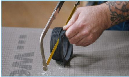
Make a cut within one of the cutting grooves to adjust the extension to the height needed. Leave the extension a bit longer than needed (by one cutting groove). The Drain Cover Extension should connect to the threaded Alignment Ring 1 securely and for good support, which requires at least one full turn of the extension's male threads reaching into the Alignment Ring 1's female threaded part.
