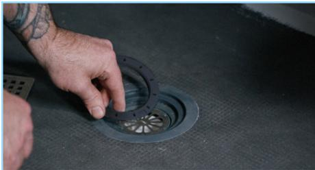
Loosely insert Alignment Ring 1, aligning with the arrow printed on the drain unit. Alignment Ring 1 has a threaded inside which will later allow you to insert a Drain Cover Extension. This piece also has built in drainage slits to allow the thinset mortar around the drain area to drain water more quickly.
