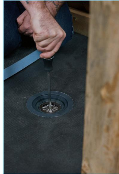
Insert a flat headed screwdriver into the Strainer Key slit and turn **LEFT** to tighten the compression seal (turn Counter-Clockwise). Achieve a hand-tight fit and **do not over-tighten**.
