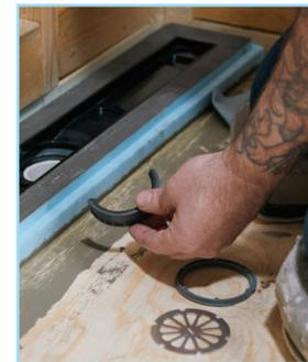
For linear drains, use a sharp utility knife to cut the compression spacer into two halves along the pre-made cut lines/notches. This will allow you to insert both halves through the the narrow drain opening. **Note:** The rubberized part of the Compression Spacer is not part of the wedi drain's waterproofing design – it is used solely to keep all dirt out of the drain connections.
