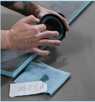
wedi provides a safe lubricant packaged with each Fundo Click and Seal™ drain component. Be sure to always use the lubricant on all rubber parts in the assembly. Lubricant packaging may vary.
