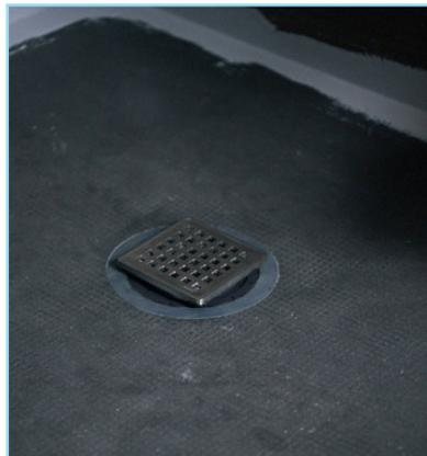
Point drain cover units can be moved  $\frac{3}{16}$  of an inch in any direction during tiling to allow for a perfect alignment and final positioning and is always fully supported, even after height extension. The cover itself can also be rotated for alignment with tile. The Fundo Click and Seal™ drain installation is now complete!
