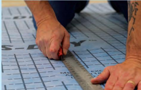
Cut wedi® S-DRY™ membrane to size prior to mixing of thinset adhesive using scissors or a utility knife.
