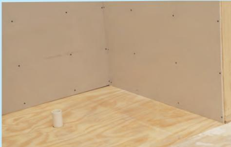
Subfloor is stable and load bearing, flat and level, and meets deflection criteria of minimum L/360 as per IRC. Wooden or concrete structural substrates are dry and sufficiently load bearing considering live and dead load.
