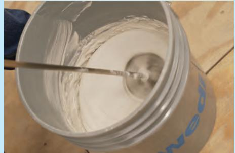
Naturally tapered drywall seams should be prepared using wedi® PRO-SET™ or appropriate patching material to ensure finished membrane is installed over flat substrate.
