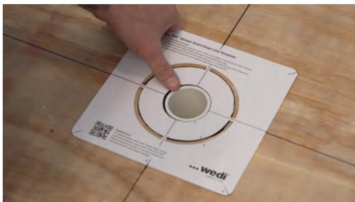
Easy to connect to waste pipes cut flush to the sub floor surface using the wedi® S-DRY™ Shower Drain/Slope line template.
