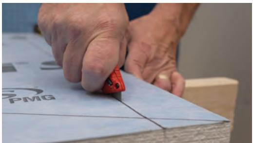
The cutting of the S-DRY™ base is done with just a utility knife and straight edge and is dust free. The bases are oversized for flexibility.
