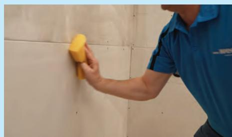
If drywall seams are covered with drywall compound, a PVA primer must be used before installing wedi® S-DRY™ Membrane. If no compound is present, use a moist sponge to wet drywall or CBU.
