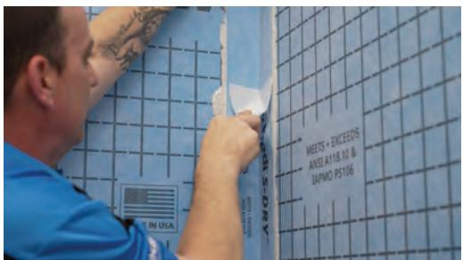
Wall membrane installation can be done with wedi® S-DRY™ and wedi® S-DRY™ XL. Seams can be taped or overlapped and actively waterproofed and bonded with wedi® S-DRY™ SEAL.
