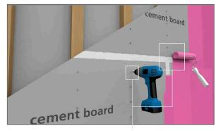
The need for thinset applied mesh tape and applied waterproofing is time consuming, messy and it is difficult to achieve a uniform waterproofing covering the full surface without leaving pinholes.
