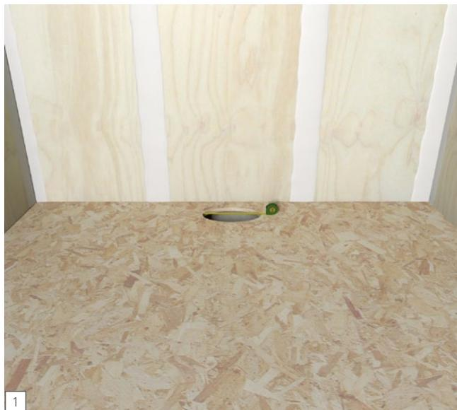
**EN** Cut the 2" (50.8 mm) pipe 1 1/4" (31.8 mm) below the top of the Subfloor. Use the oval shape cutting template where you want to position the drain to cut out subfloor using a jigsaw to allow wedi drain trap to be inserted and connected to floor pipe using appropriate ABS compatible or multipurpose cement glue. Please also check cement glue compatibility to floor pipe material. The drain and trap have to be secured to the subfloor. Drain recess cut out must not add deflection to subfloor.
