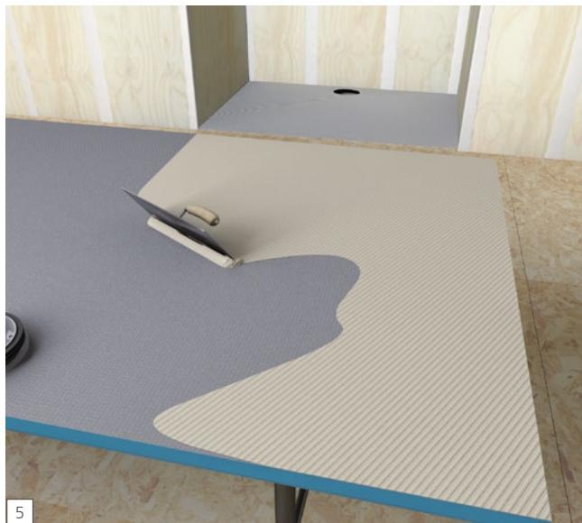
**EN** Trowel the thinset on the rear side of the Fundo again using a 1/4" x 1/4" (6.4 x 6.4 mm) notch trowel.
