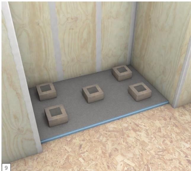
**EN** Press the Fundo firmly into the thinset bed, ensuring that the installation is level and void free. Apply some weight equally and leave on surface and drain area to allow the thinset to initially cure without being disturbed (e.g. thinset bags).
