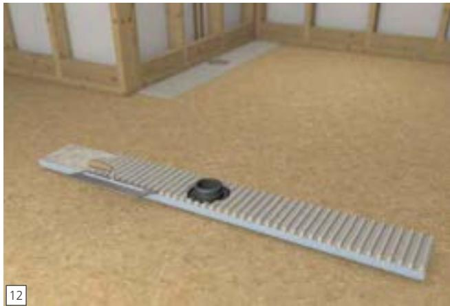
**EN** Trowel the thinset on the rear side of the Fundo again using a 1/4 in. x 1/4 in. notched trowel. Flat trowel the thinset over the entire product's cement surface, then comb through thinset bed creating channels pointing in same direction as applied on subfloor.
