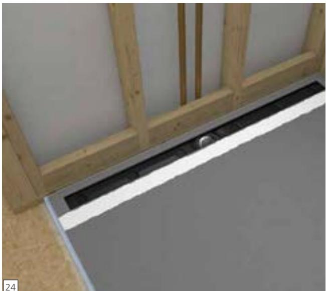
**EN** Trowel flat all excess sealant. Another 1/2 in. bead of wedi joint sealant is applied over and along the connection seam later (to avoid large areas with fresh sealant covered seams during the installation phase).
