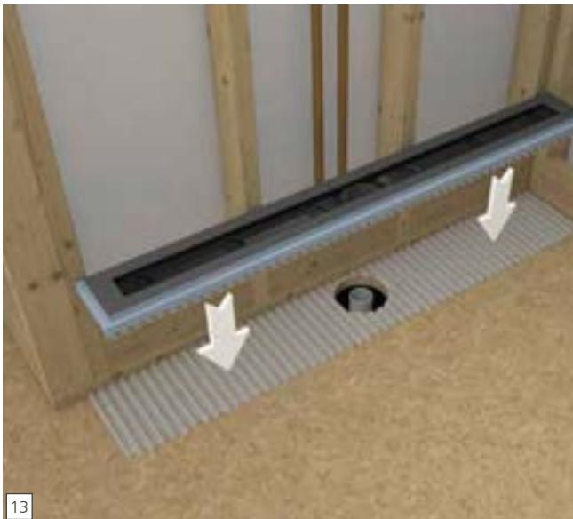
**EN** Place the Fundo Riolito line module into the thinset bed and press firmly into resting position and ensuring full coverage of thinset mortar between line module and subfloor leaving no voids. Ensure floor waste pipe is centered within Fundo Click and Seal drain unit. Ensure line module is squared up tightly with wall framing and is coming to rest in a level position. Apply some tile boxes/weight to keep the thinset mortar compressed during initial drying.
