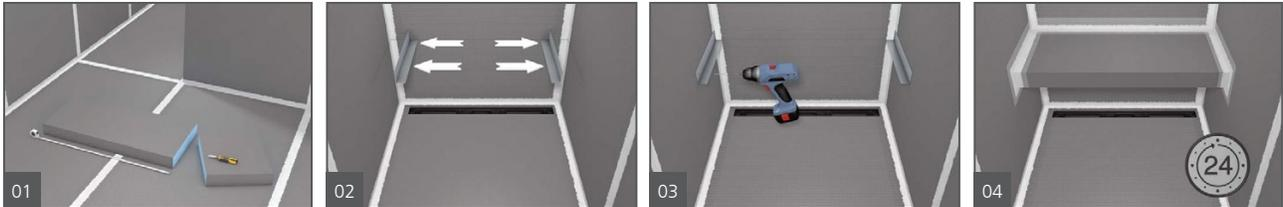
1. Cut and dry-fit the bench into the three-wall opening in the shower. Dry-fit with the two L-shaped steel profiles loosely fitted onto the sides of the bench. Mark the outline of the bench where it will connect to the walls so you can see later where to apply wedi® Joint Sealant.
