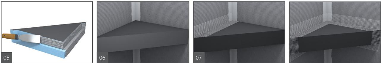
5. Press the seat element into position and apply a weight (i.e. tile box) so the sealant can set under bond pressure.
