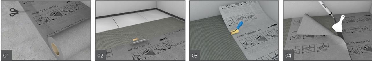
1. Lay out wedi® Subliner Dry and cut to size using a knife or scissors.
