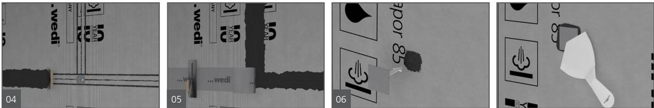
4. Apply several beads of wedi® Sealant 620 as a setting and sealing bed for wedi sealing tape. Spread the sealant with a fine tooth adhesive trowel or flat putty knife to achieve a full coverage sealant bed for the sealing tape. The minimum thickness of the sealant bed should be 1/16 in.
