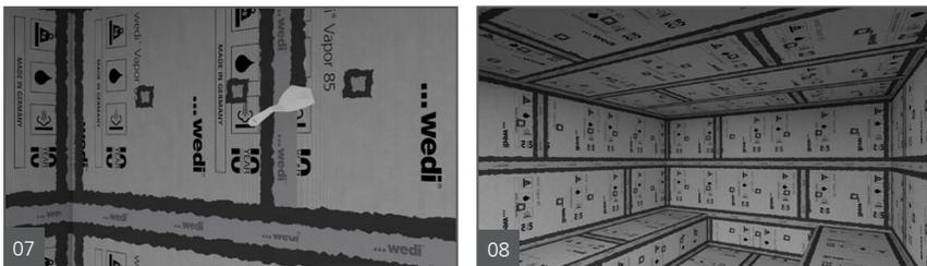
7. Use wedi® Sealant 620 and wedi® Subliner sealing tape and sealing collars to seal around protrusions and penetrations of the Vapor 85 using the same method as for applying tape and fastener point covers. If you can't clearly see Sealant 620 past the perimeter of 5 in. tape once it is embedded in all areas of the application, a bead of
